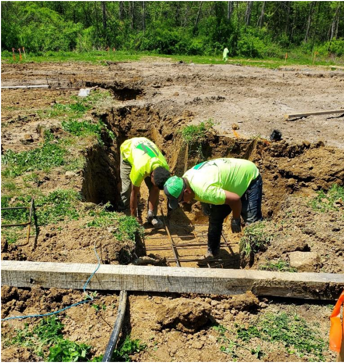
Picnic Pavilion Footers Being Prepped AJ Asphalt May 9th
