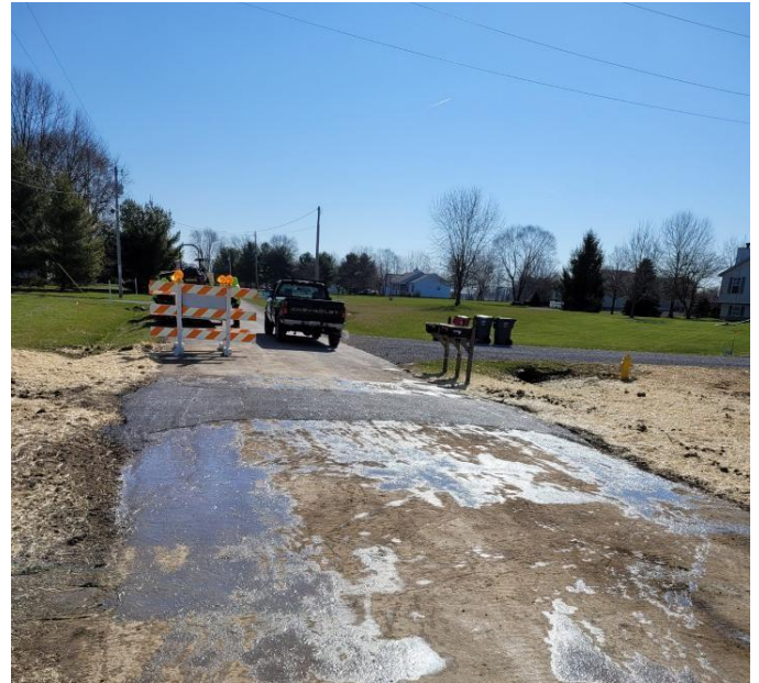
Todd Street Road Culvert Installation
